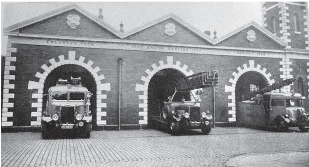
Old Preston Firestation, Tithebarn Street, Preston. Courtesy of Preston Digital Archive.
